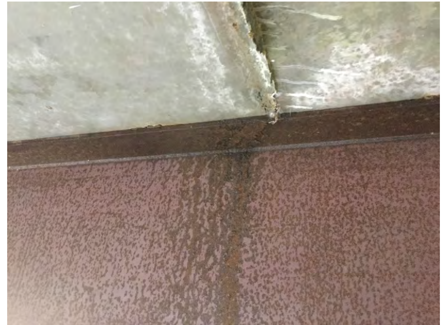
Indications of deck joint condition
