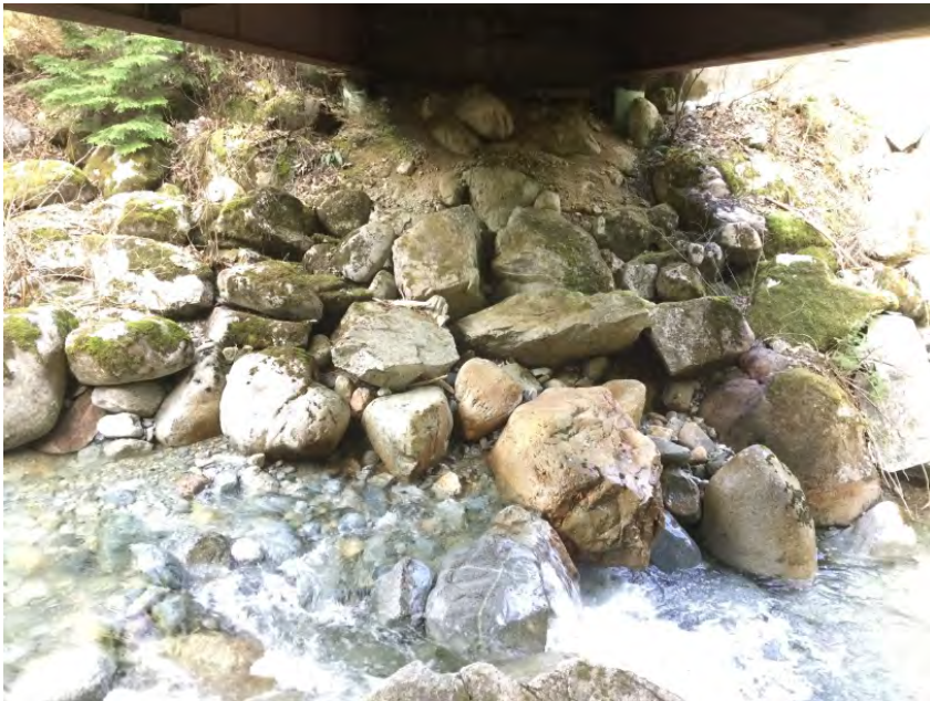
Left Bank Abutment when facing downstream
